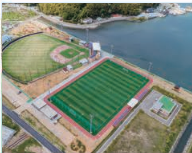
Ha cheong Sports Town Baseball Ground, Football Ground
