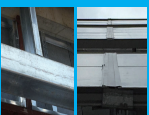
Project photo - staggered panel joint
