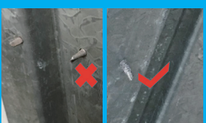
Project photo - ineffective self tapping screw
